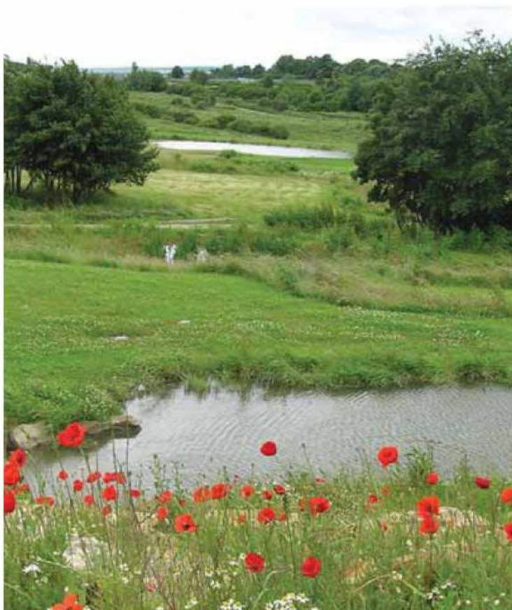
Figure Q: SuDS detention basins serving social housing developments on the Manor Estate in Sheffield
